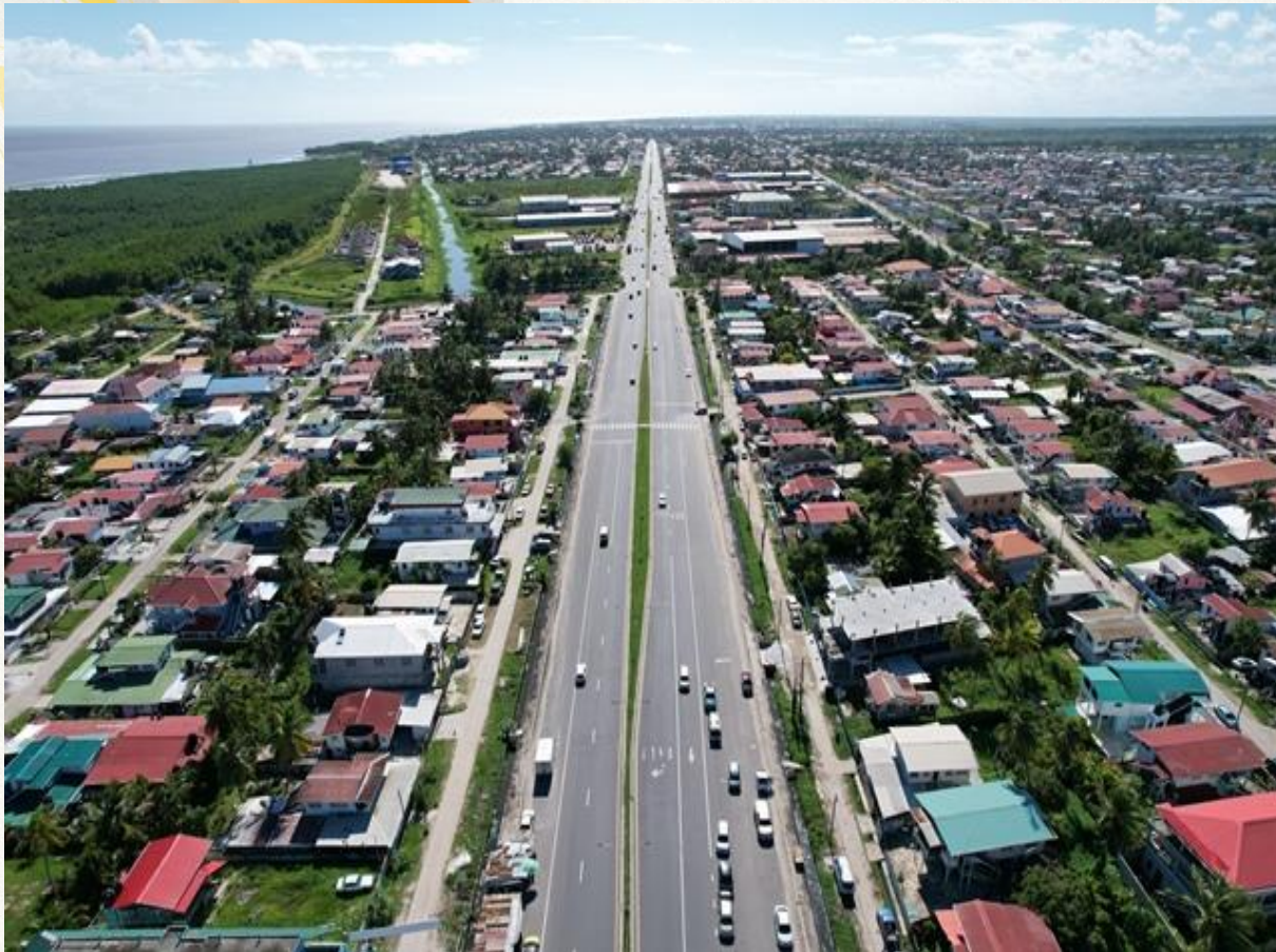
Construction of Phase I East Bank – East Coast Road Linkage Project, Guyana
