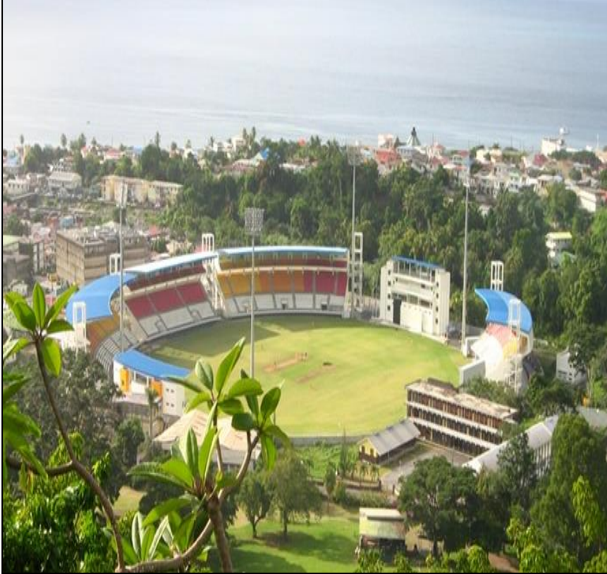
Construction of Cricket Stadium at Georgetown under Exim Bank's GOI-supported Line of Credit to the Government of Guyana .
